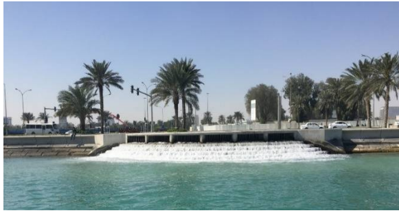
Figure 5. Doha Corniche large water outlets.
