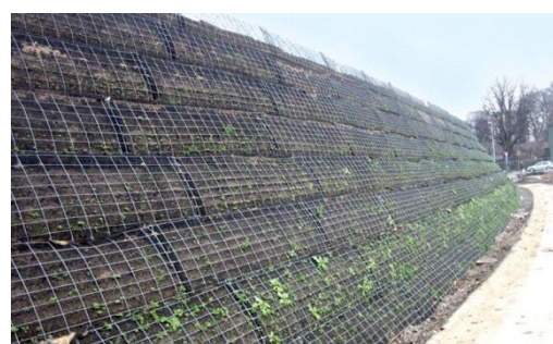
Fig.6. Combination geogrid reinforcing with gabions
