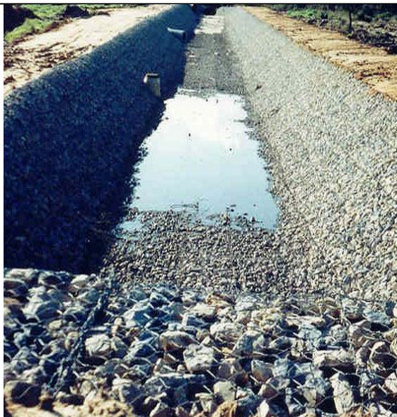
Fig.3. Channel coating for preventing erosion with gabion mattresses.
