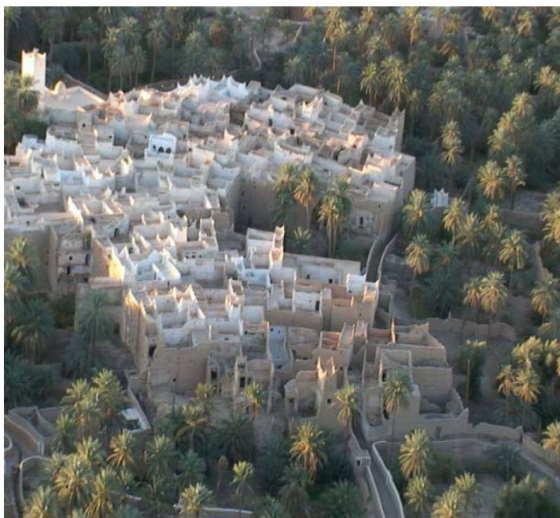
(Figure 2) The Oasis of Ghadames, the capital of the Libyan Desert. An example of the architecture of desert oases, with traditional compact fabric and the unity of the residential Neighborhood Source: Mirathlibya.blogspot, 2/7/2012
