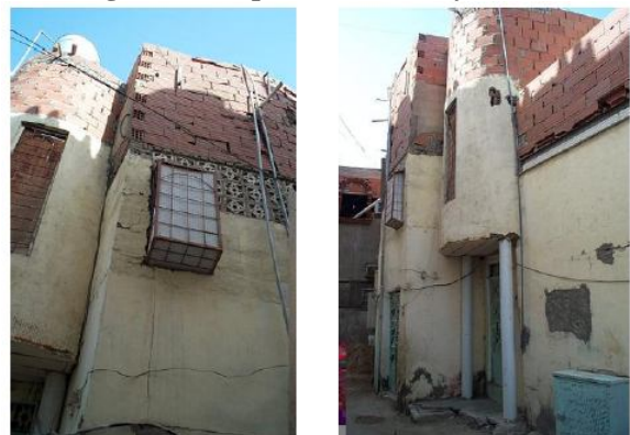
Fig. 11. Cement bricks and steel used in the construction of al-Sabeel dwellings (Source: pictures taken by the author)
